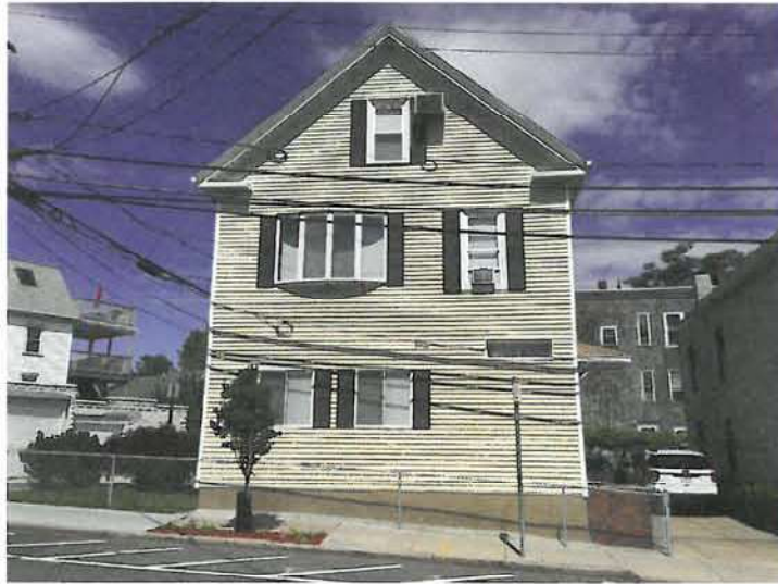
East Side of Dane Street
